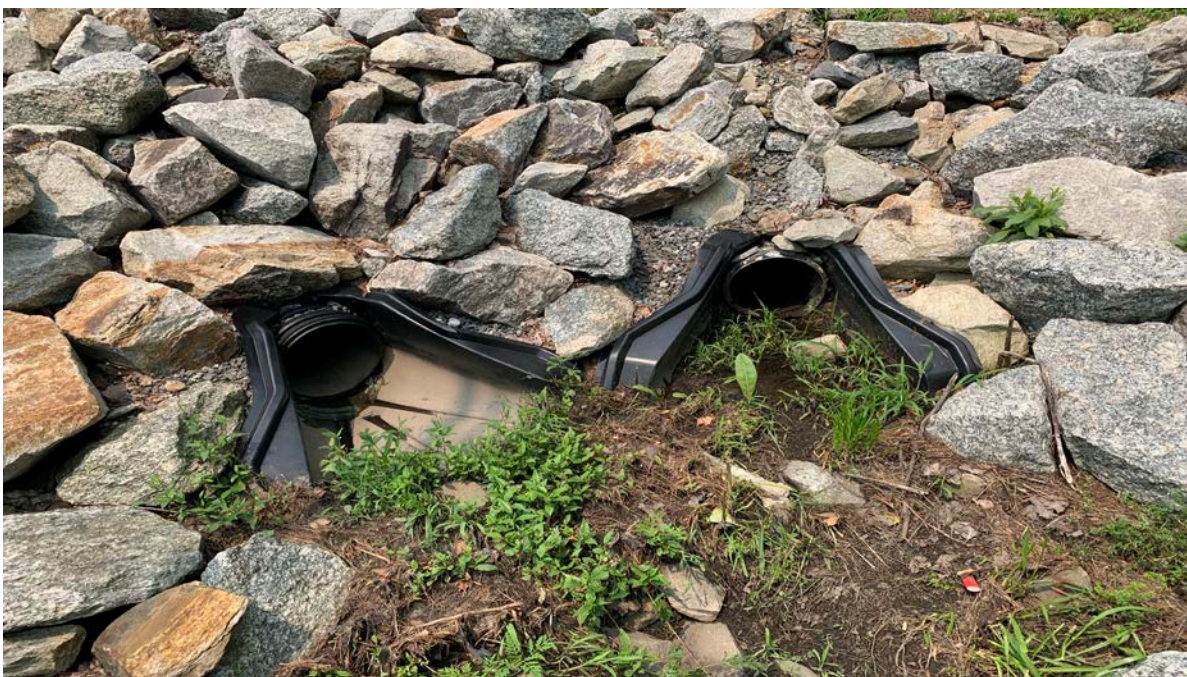
Photograph 10: Left downstream channel slope. Photo shows discharge (left flared end) location of 2 left most catch basins on Lake Road that drain to the downstream side of the dam and through the left channel slope. The flared end shown to the right is the discharge location from a catch basin located further up Lake Road to the left of the dam. Pipes are a 12" HDPE (left) and a 12" CMP (right).
