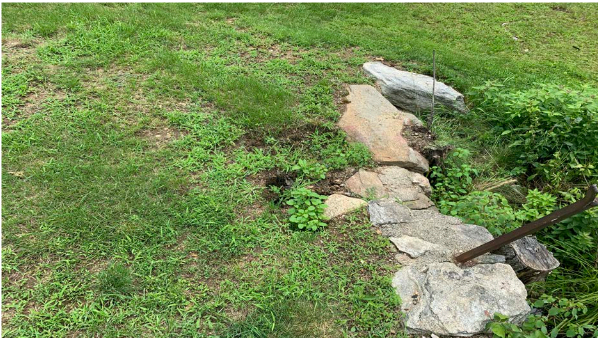
Photograph 4: Right upstream stone masonry wall and embankment. A small sunken area was observed behind the upstream stone masonry wall to the right of the spillway.
