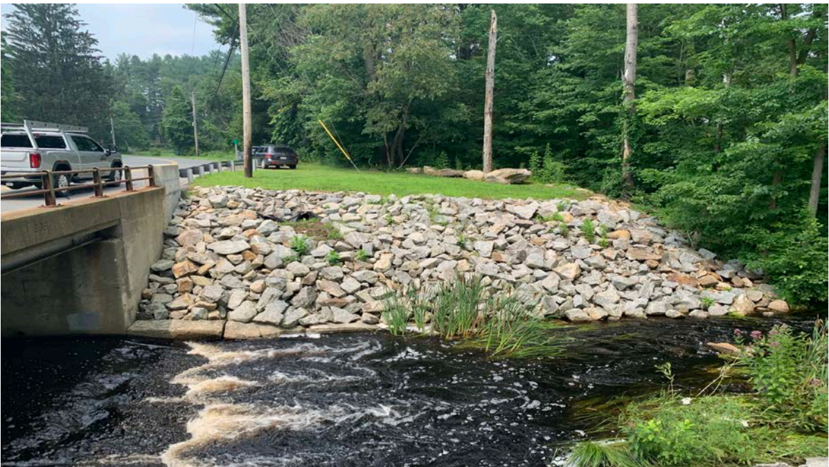
Photograph 8: Left downstream dam embankment and channel slope. A gravel parking area was located on the earthen embankment near the left abutment.
