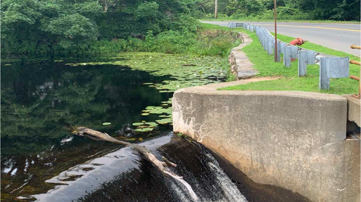
Photograph 13: Left spillway training wall/bridge abutment. Some minor cracking was observed in the left concrete training wall/bridge abutment.
