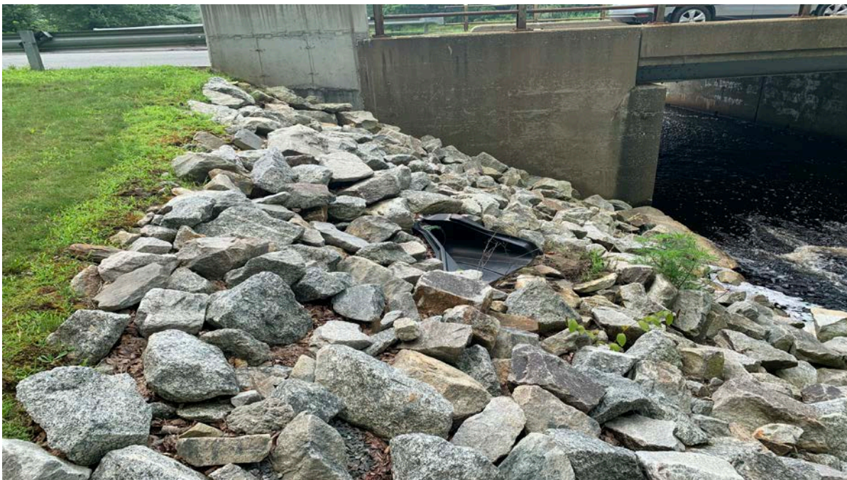
Photograph 11: Right downstream channel slope. Photo shows discharge location of 2 right most catch basins on Lake Road that drain to the downstream side of the dam and through the right channel slope. Pipe is a 12" HDPE
