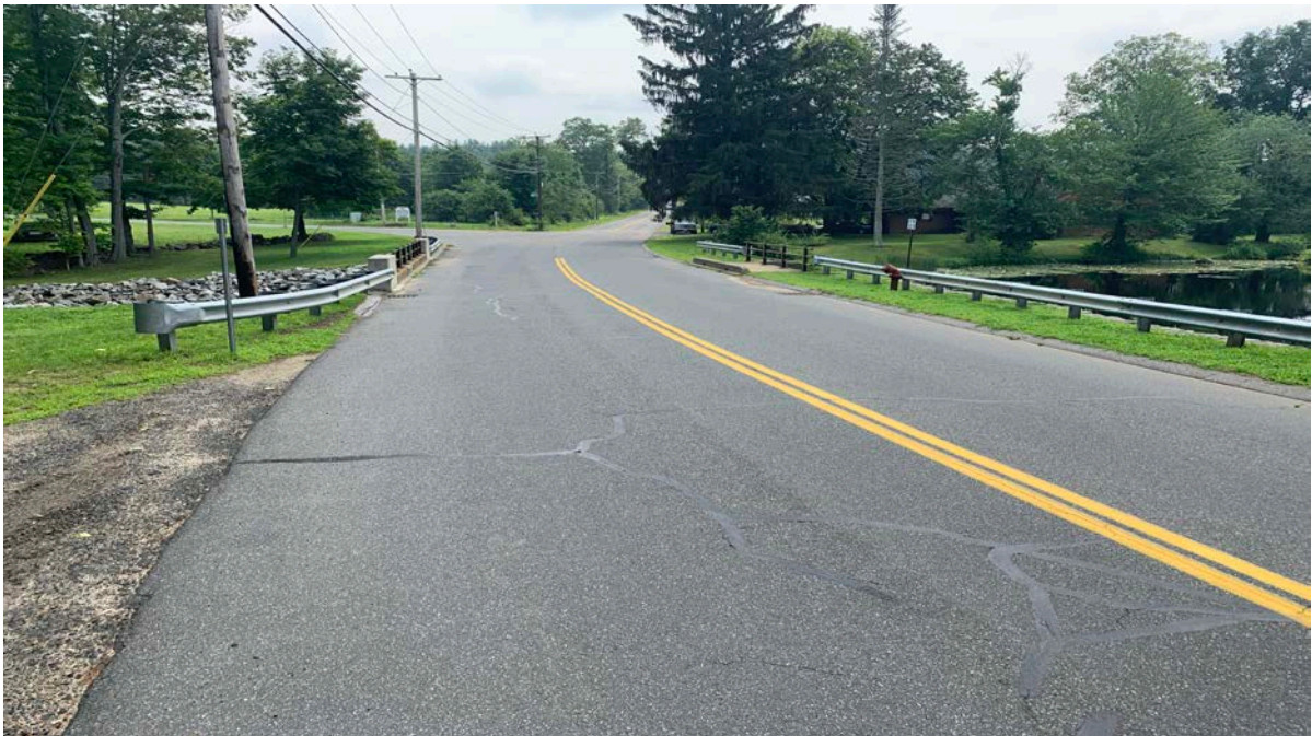
Photograph 6: Minor cracking was observed in the asphalt paved crest. Photo was taken from the left abutment to the right abutment.
