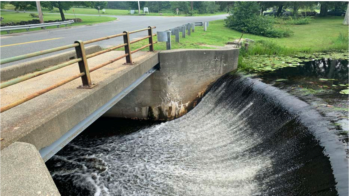
Photograph 14: Right spillway training wall/bridge abutment. Some minor cracking was observed in the right concrete training wall/bridge abutment.
