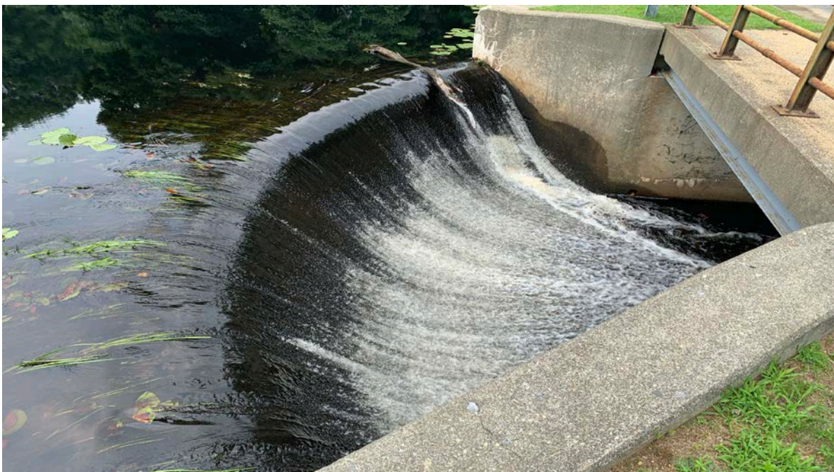
Photograph 12: Spillway ogee weir from right crest embankment. Minor debris was observed at the spillway crest.
