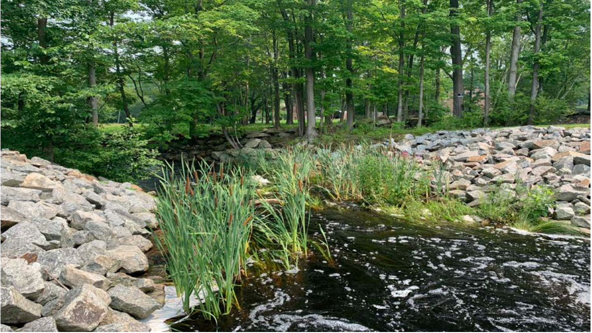
Photograph 15: Downstream area. Vegetation is growing within the channel.
