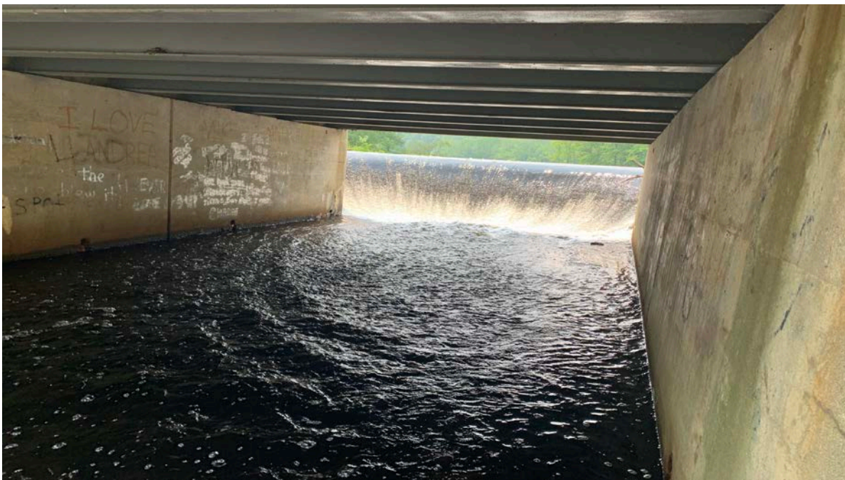
Photograph 9: View under bridge from downstream side. Weep holes were observed at the base of the bridge abutments that also serve as the spillway training walls.
