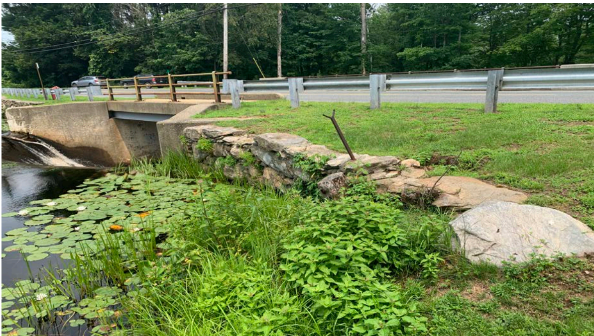
Photograph 3: Right upstream stone masonry wall and embankment. The right upstream stone masonry wall was missing stones at its base and along its top and was leaning outward toward the impoundment. There was some minor brush growing through the wall.
