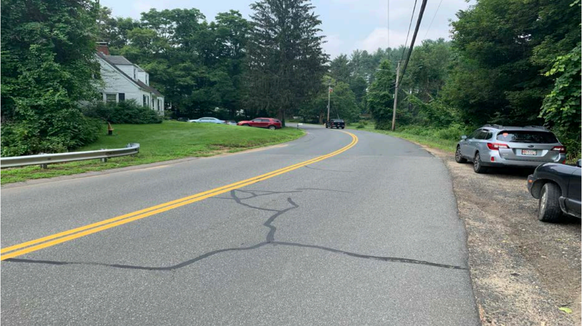
Photograph 1: Left abutment viewed from the crest. Lake Road passes directly over the left abutment.
