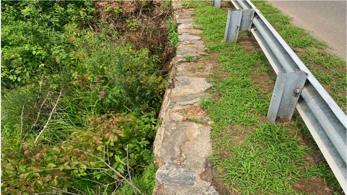
Photograph 5: Left upstream stone masonry wall looking toward the left abutment. The wall was missing cap stones in multiple areas.
